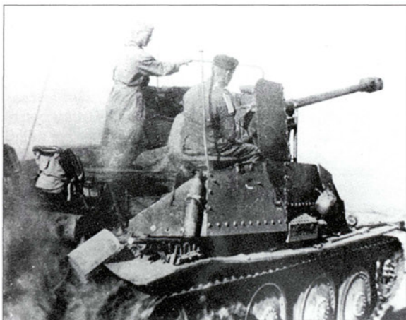
The captured Russian 76.2mm anti-tank gun was rechambered to take German 75mm rounds, and mounted on the chassis of the obsolete Czech 38t to produce the Marder III. In May 1942, 117 of these vehicles were sent to North Africa to counter the menace of the heavily armoured Matilda II. (Bundesarchiv)
